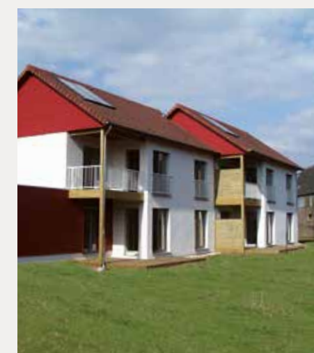
↓ Chauffe-eau solaire individuel, En-Act, Architecture, Les Airlles
